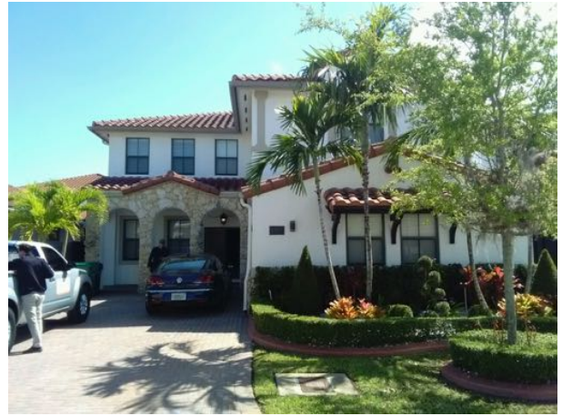
All Exterior Openings Are Impact Rated
