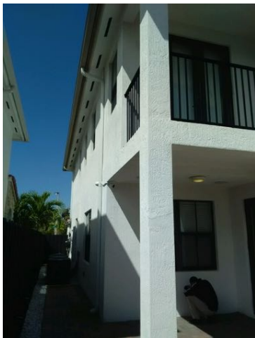
All Exterior Openings Are Impact Rated
